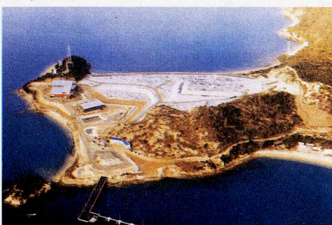
Site picture after the provisional measures for the conservation of the environment has been completed
