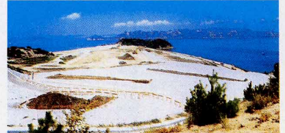
Covering the air-transmission sheet
